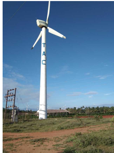
5 x 225kW WINDFARM
